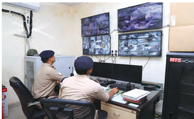
CCTV surveillance control room
